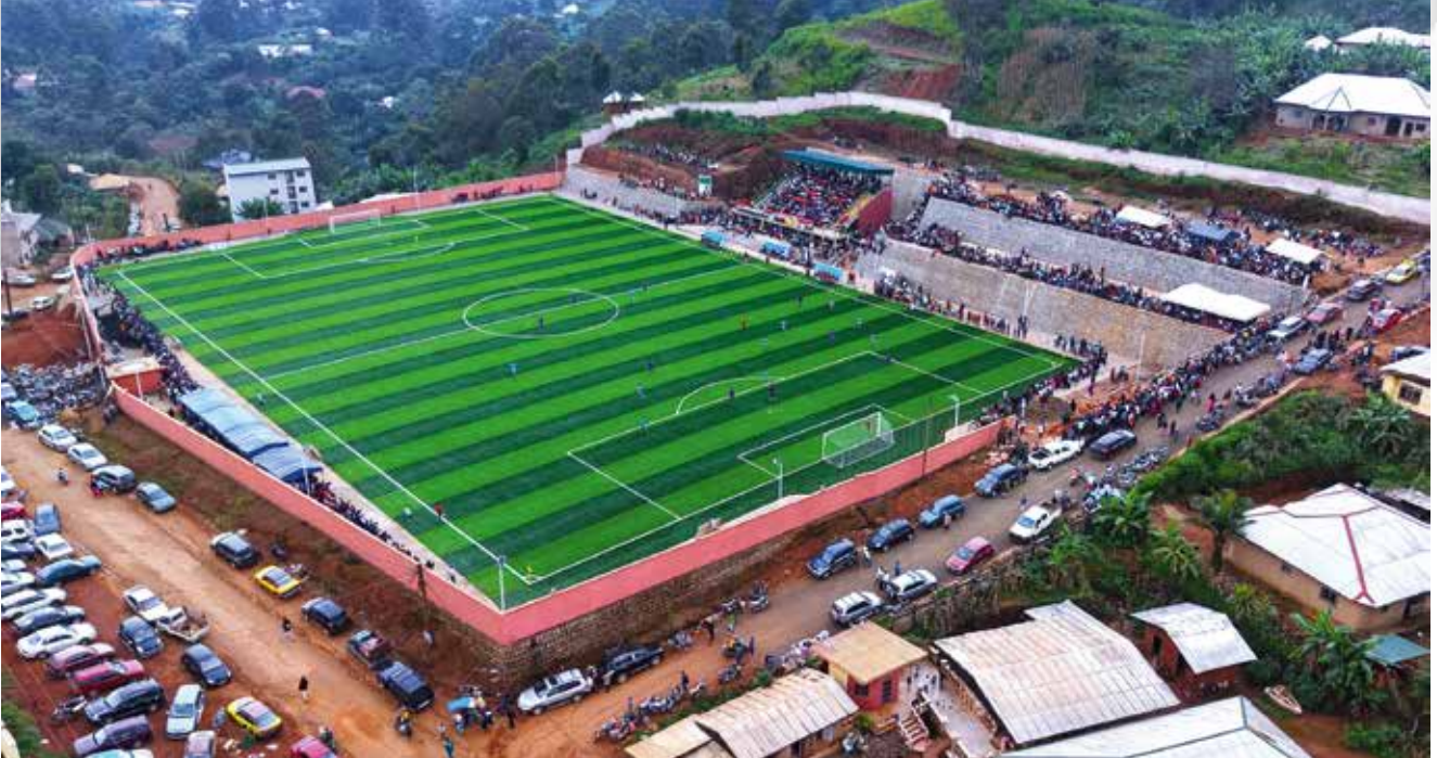
Aerial view of the Bamenda Proximity Stadium
