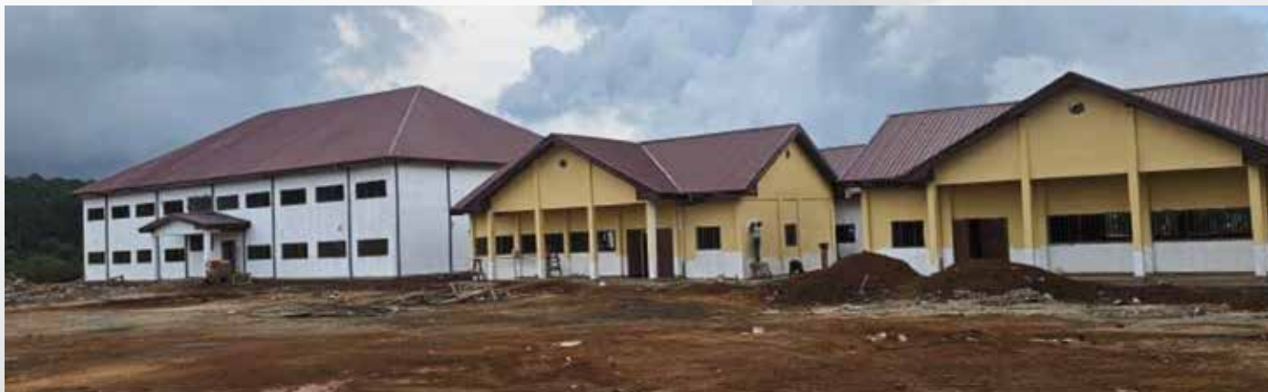
Construction and equipping of GTHS NKAMBE, Work Progressas at April 2026
