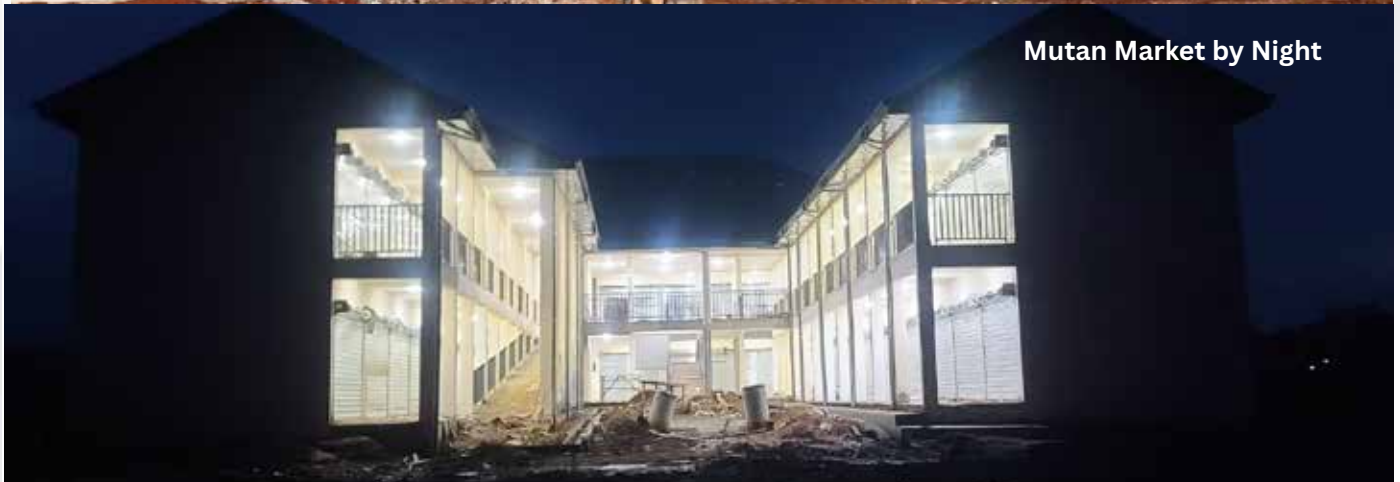
Construction of Mutan Market in Bamenda, Mile 6 Nkwen.
