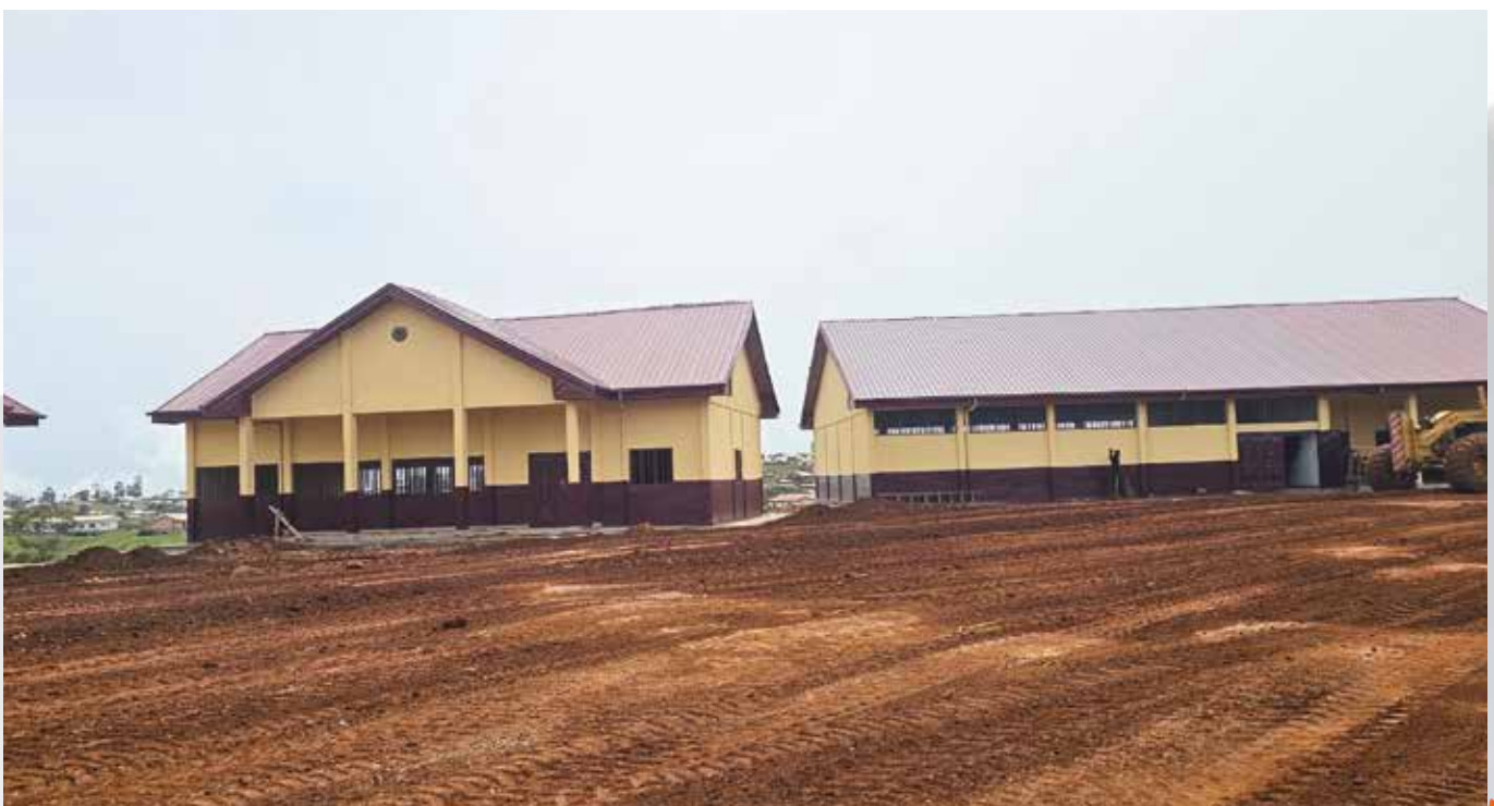
Cconstruction of GTHS Nkambe (PROLOG Project)
