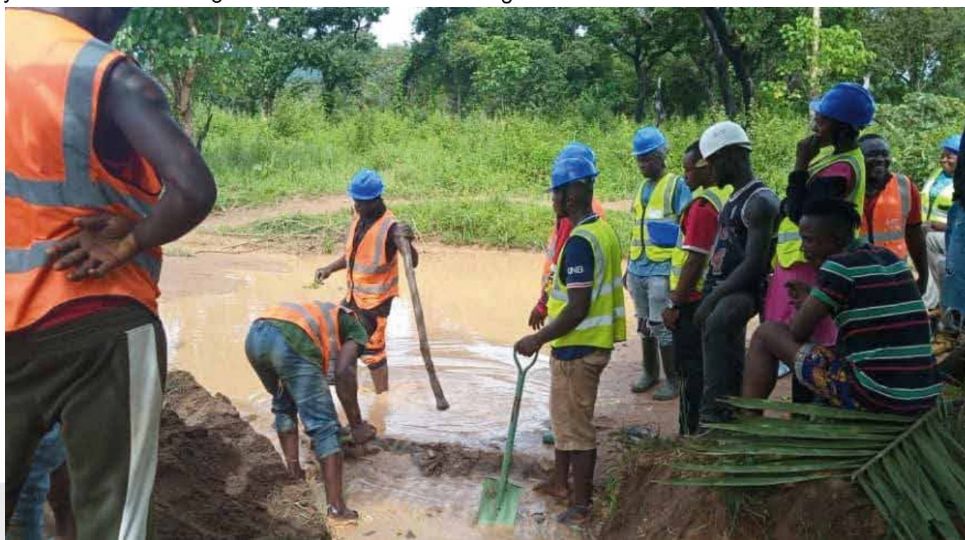
The Manual maintenance of the AKO - DUMBO BERABE road (PDI)
