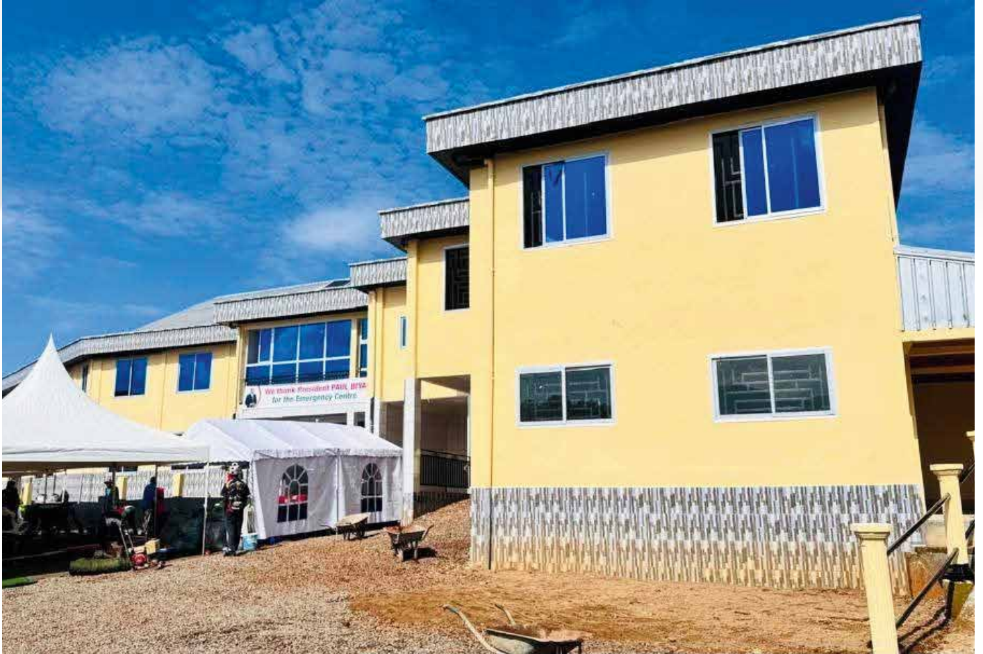
Construction of Emergency Centre at the Bamenda Regional Hospital
