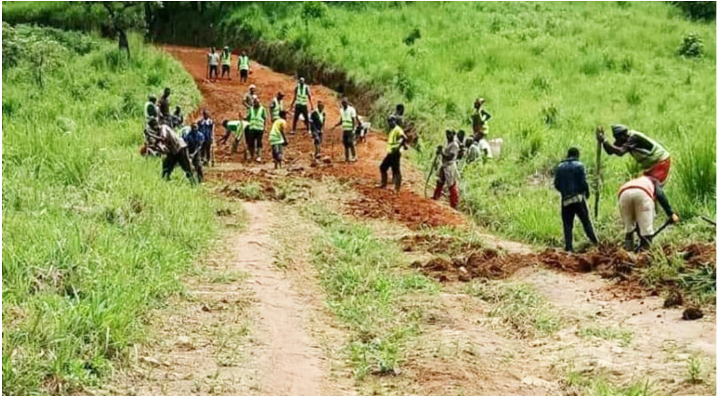
Road works for the Regional Assembly's PDI through High Intensive Labour Approach (HILA)- project execution in Donga-Mantung on the Nwa-Ntong road (Yamba North), Nwa Sub Division
