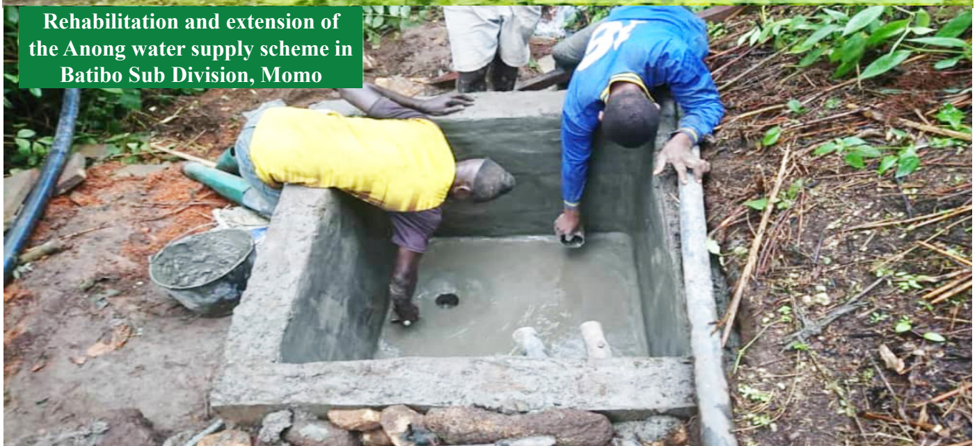
Work progress as at June 30, 2023
