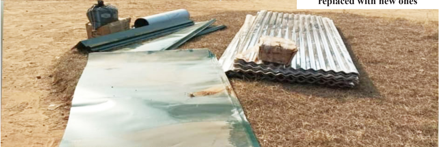
Removal of old zink sheets to be replaced with new ones
