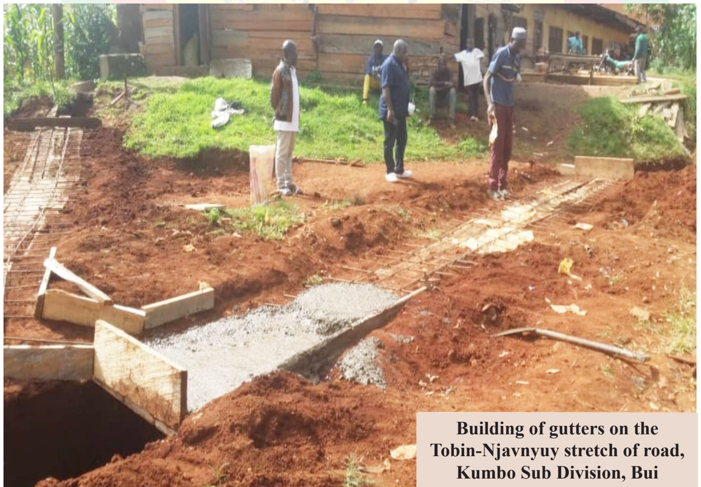
Rehabilitation of Tobin – Njavnyuy Road in Kumbo Sub Division, Bui
