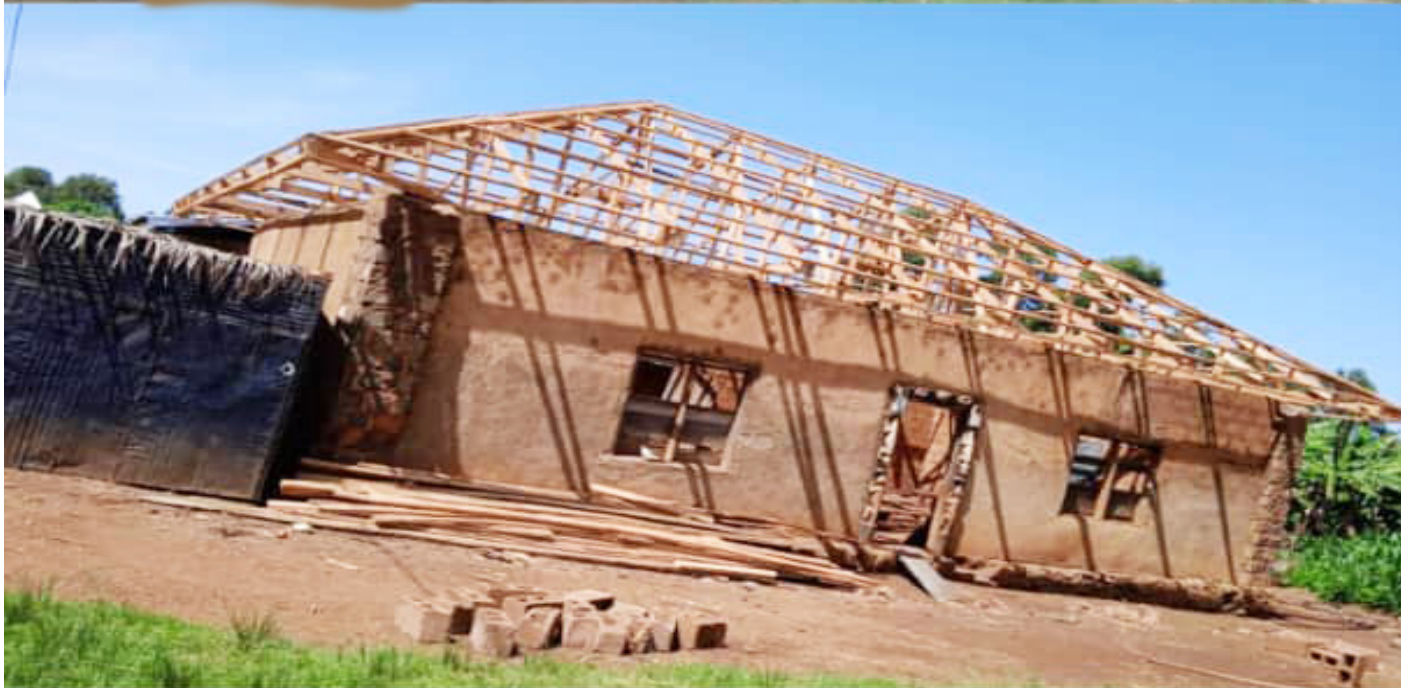
Work progress as at June 30, 2023
