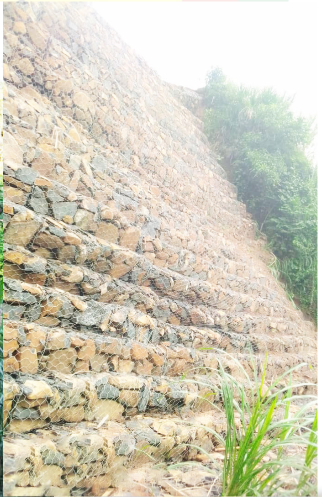
Construction of retaining wall for the rehabilitation of Regional Road (R0515) Bambui – Fundong
