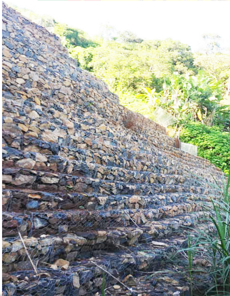
Construction of retaining wall for the rehabilitation of Regional Road (R0515) Bambui – Fundong
