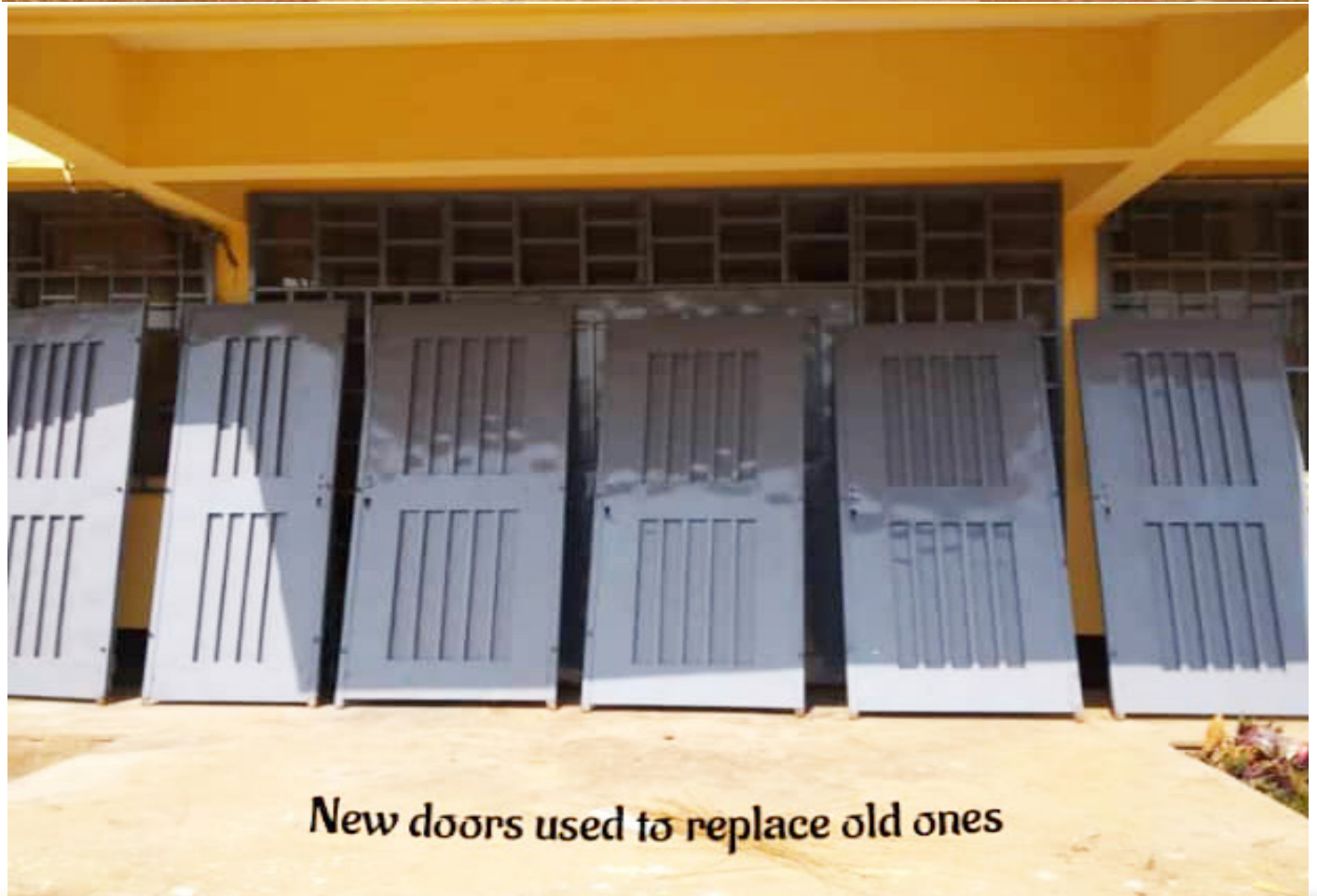
Rehabilitation of GTTC Mbengwi (Completed)
