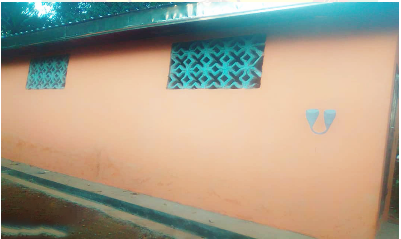
Construction of a 2-compartment VIP toilet block in Belo-Boyo Division
