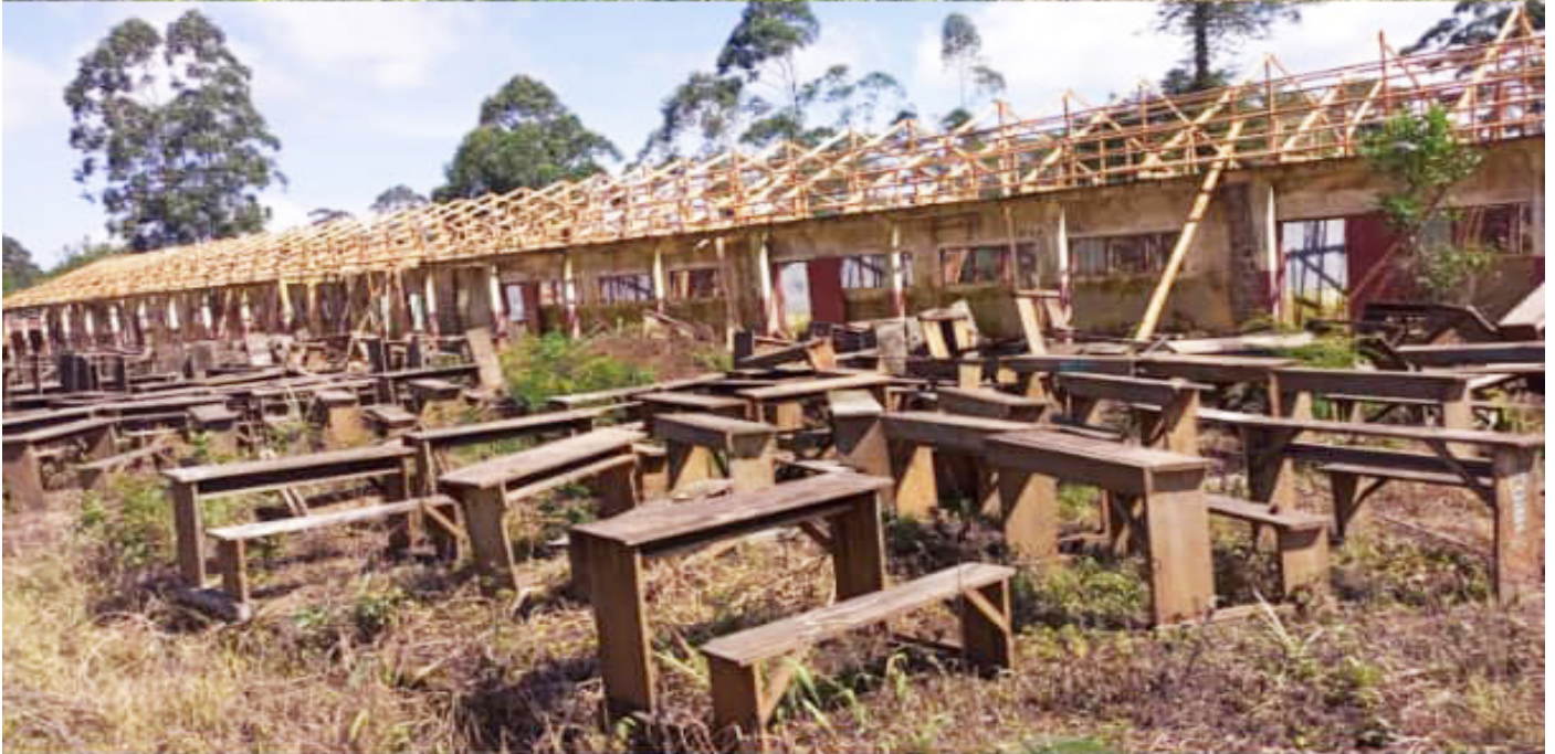
Rehabilitation of GBHS Fundong (Ongoing)
