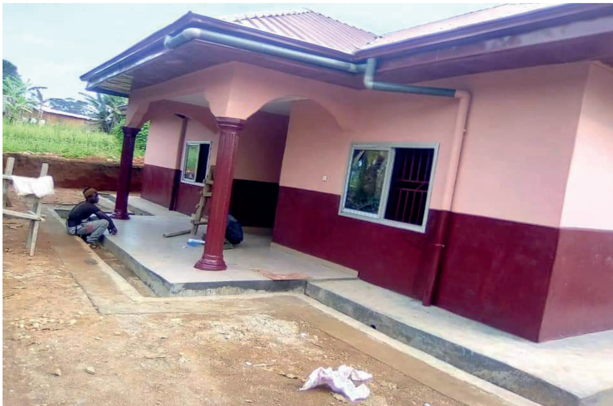
LOT 3: Construction of the Queen's Residential Quarter in Nwa
