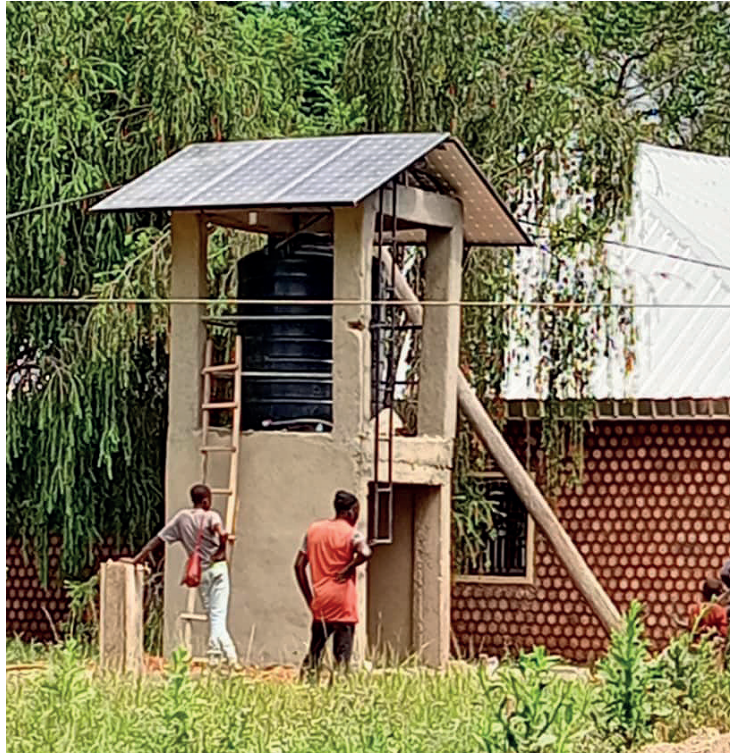
LOT 4 Water supply to palace: Borehole construction using Solar pump in Bamunka
