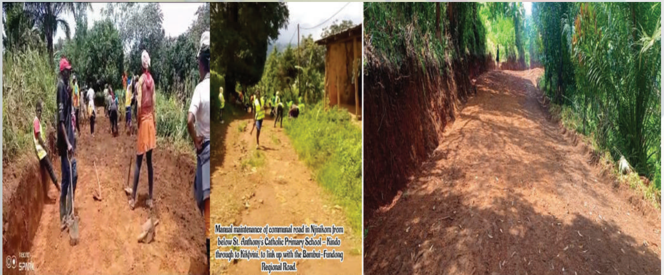
Rehabilitation of 7km road, back-filling and grubbing of gutters
