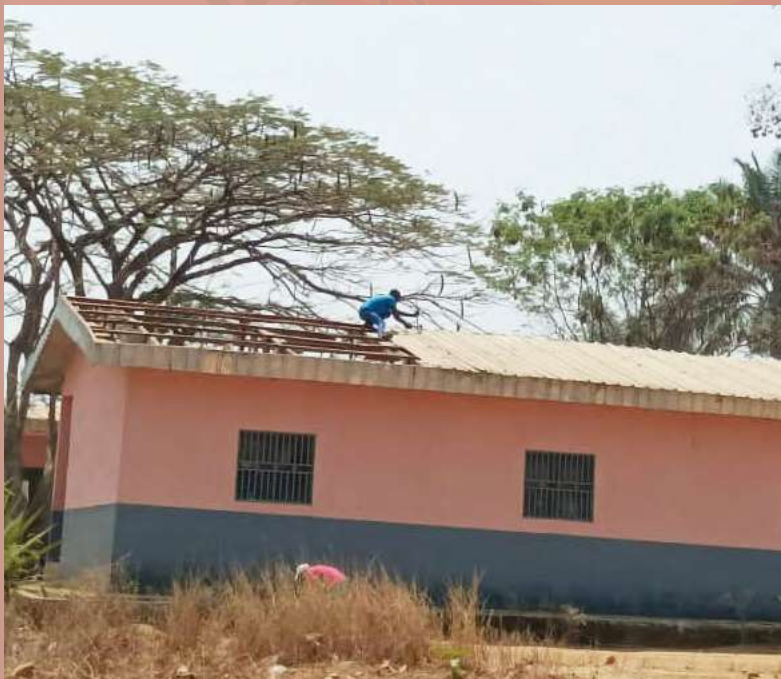
Rehabilitation of Ako District Hospital
