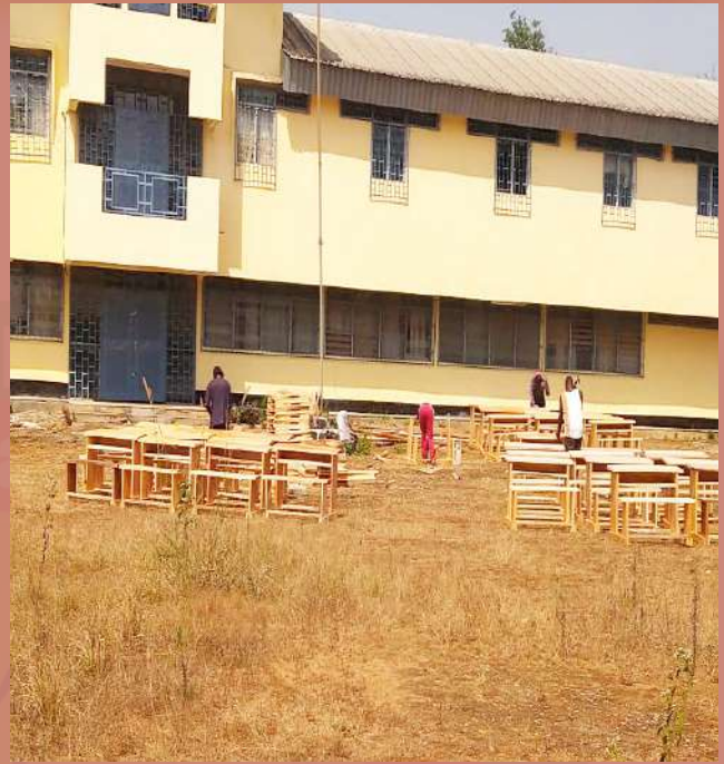
Rehabilitation of GTTTC Mbengwi
