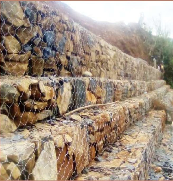
Rehabilitation of Regional road in Fundong
